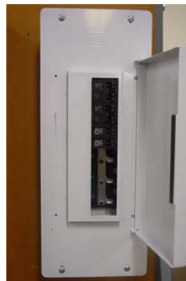
Step #3 Install New HFLCI
